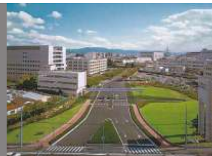
Matsushita Electric Works, Osaka
