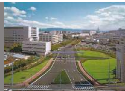
Matsushita Electric Works, Osaka
